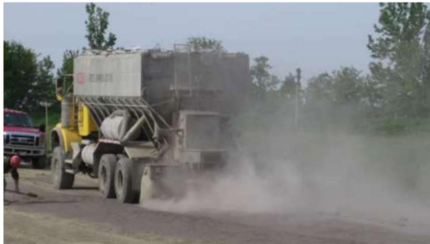
Figure 12. Spreading of the steel slag-Class-C fly ash mixture on the subgrade soil
