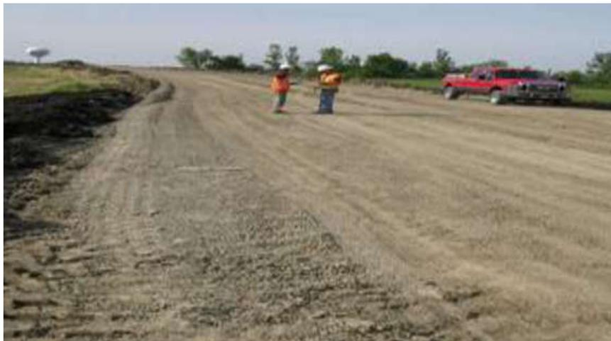
Figure 10. In situ subgrade soil of the SW ramp before soil stabilization
