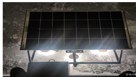
Fig 9 Led lights during night time
