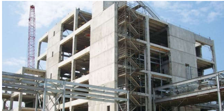
Fig-1: Shear wall building
